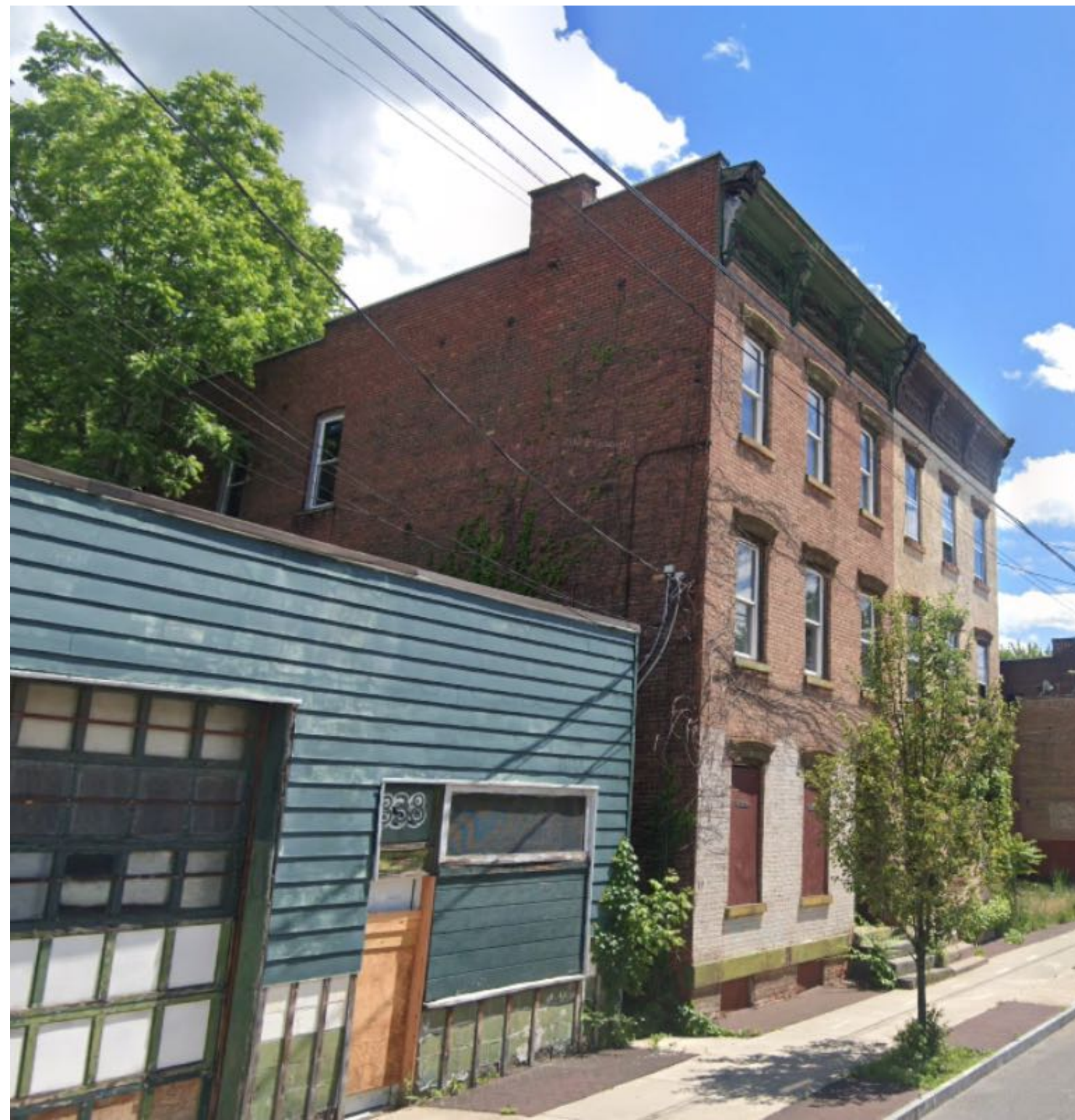
1 FRONT ELEVATION - EXISTING PHOTOS
