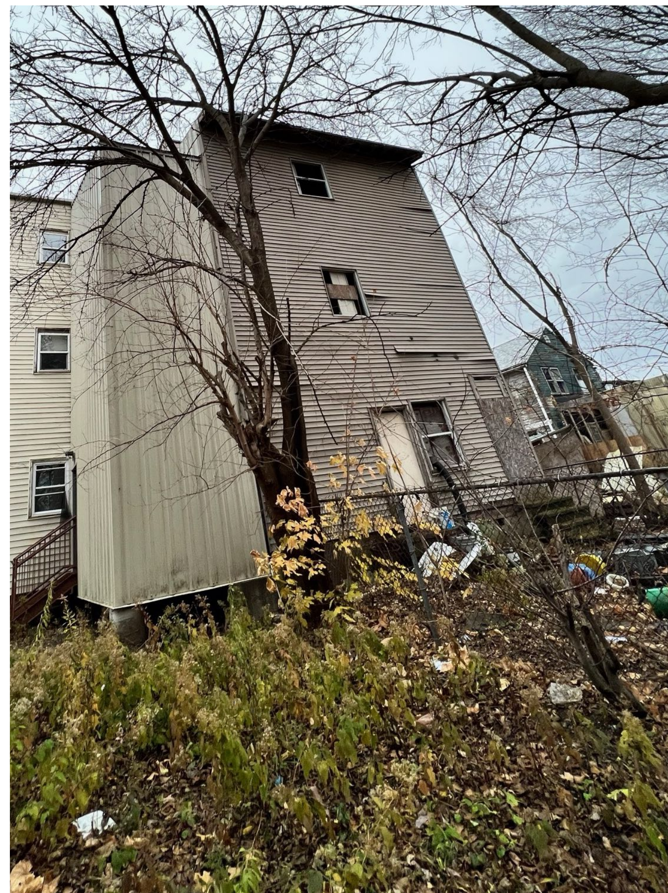
2 REAR ELEVATION - EXISTING PHOTOS
