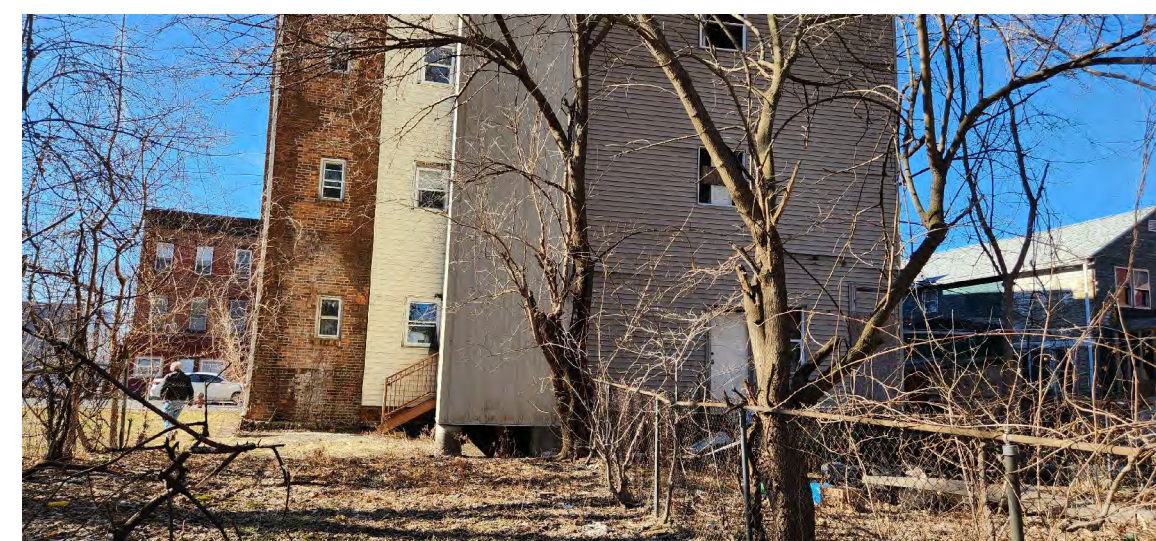
Rear Of #834 & #836 River Street
