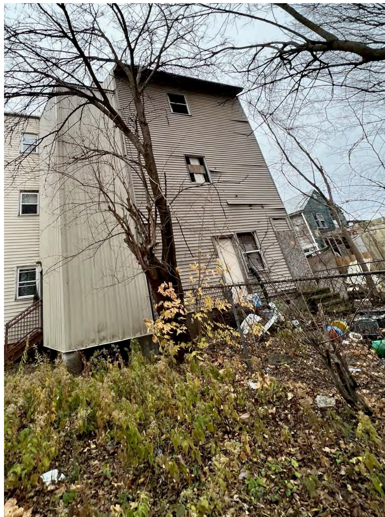
2 REAR ELEVATION - EXISTING PHOTOS
