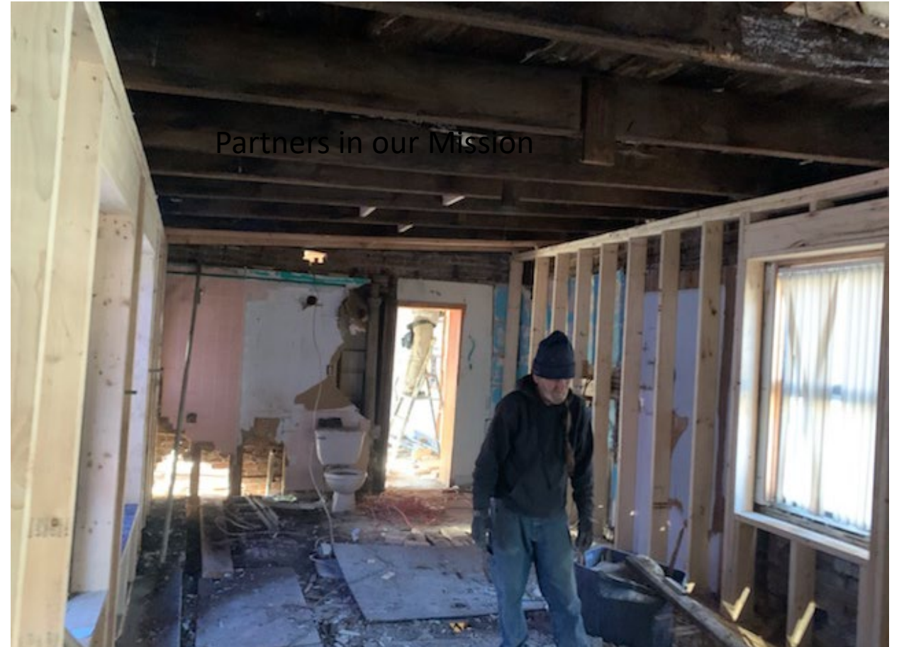
3229 6 th Ave stabilization in progress
